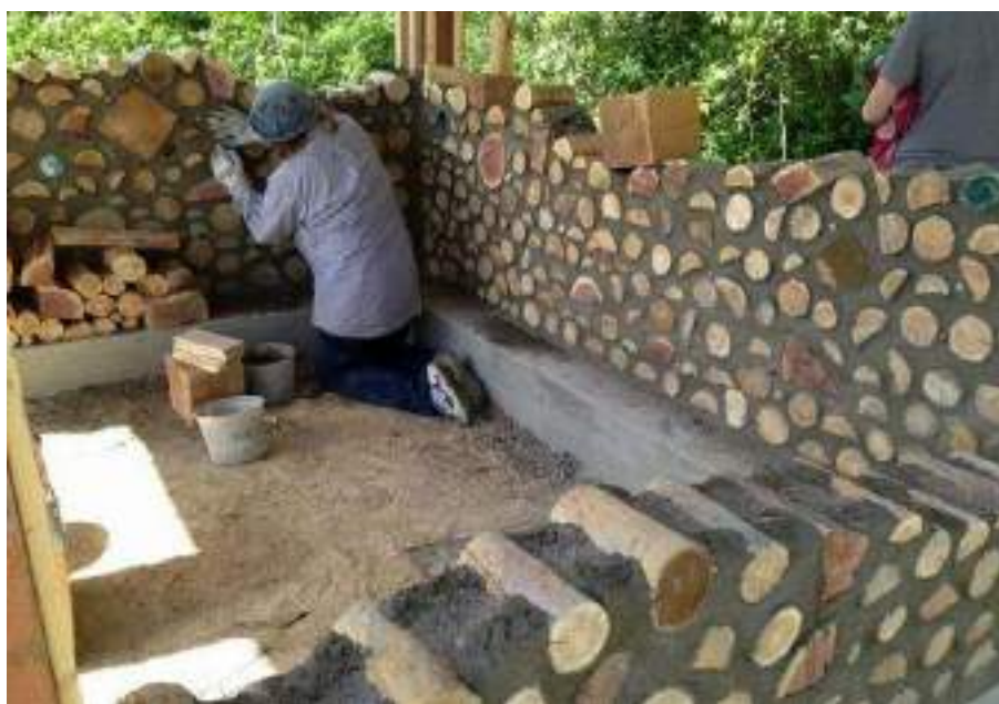
Figura 11: Parede cordwood.
